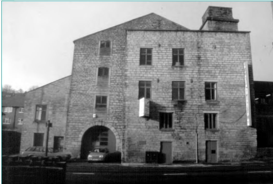
Photo 8. Textile Mill, Rossendale
